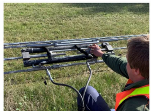
Manual checking and adjustment of cable tension
