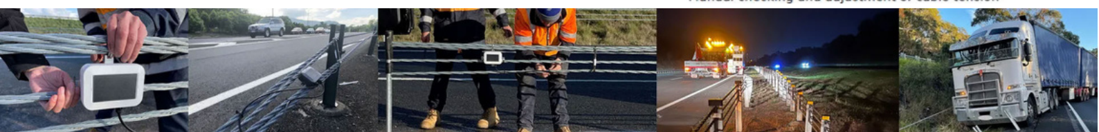
Manual checking and adjustment of cable tension
