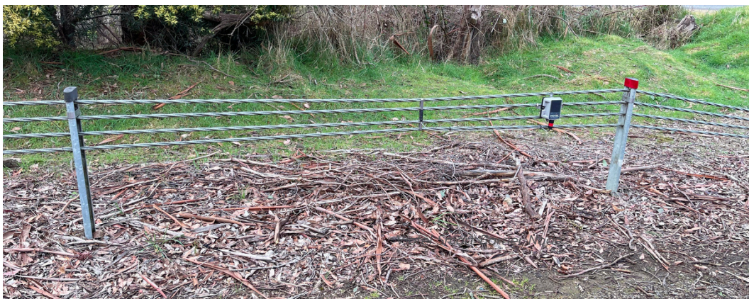
Installation on a wire rope barrier with detachable strain band
