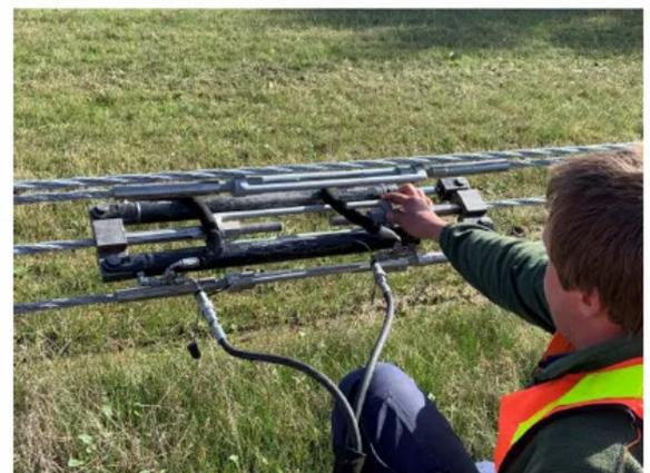
Manual checking and adjustment of cable tension
