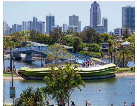
40 Million Mornings Home of the Arts (HOTA) Bridge – Gold Coast Qld. Anodised finish to custom folded panels on exterior of bridge landing
