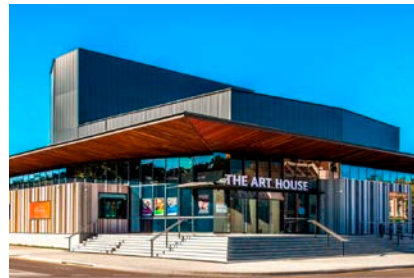
Arthouse Wyong. Anodised finish to highlight elements on exterior of building
