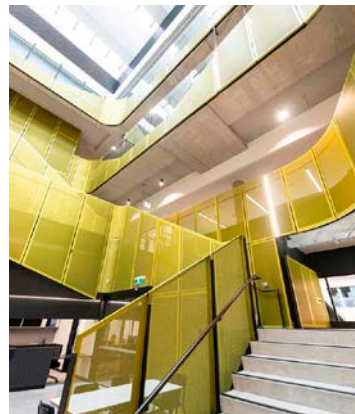
Richmond High School, Victoria. Anodised finish to perforated screens
