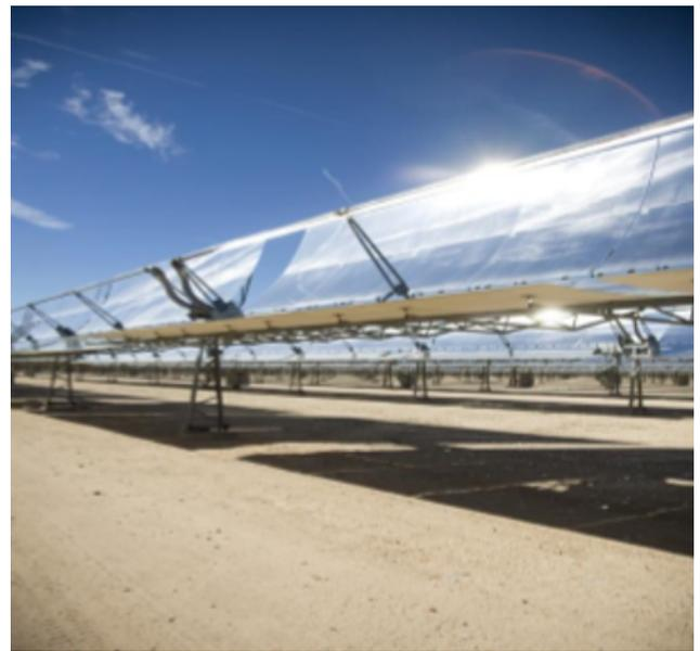
A field of parabolic trough solar collectors
