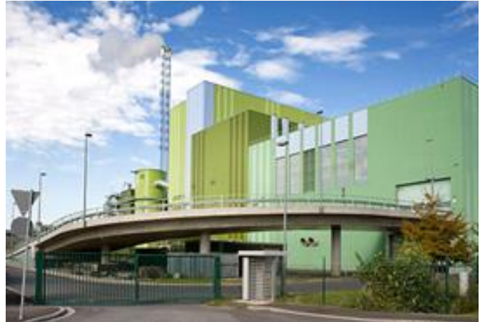
A typical EfW facility
