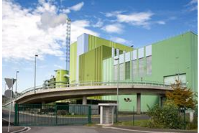
A typical EfW facility
