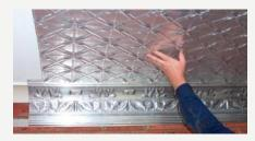
NOTE: There is no need to remove old Cornices unless the old is larger than the new. In some cases, that a batten will be needed to be fitted. Place batten correct width from the wall directly onto the ceiling, so the back of the cornice sits against it. This is to push cornice against to prevent any distortion.
