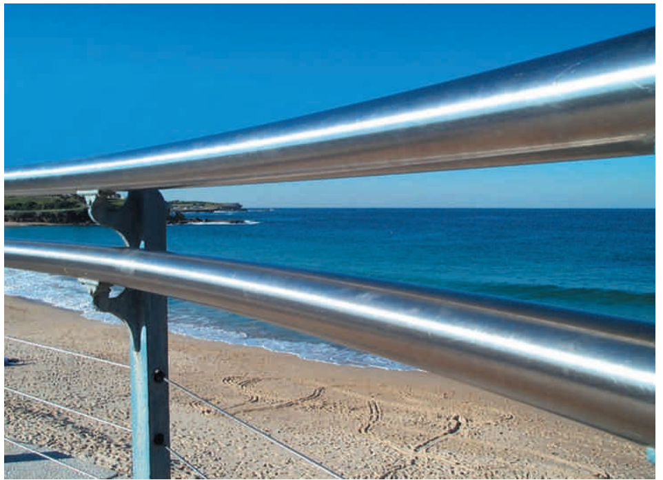
Successful use of stainless steel after more than 14 years service in a coastal environment.
