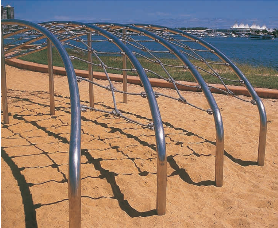
Coastal application, good surface finish — no tea staining
