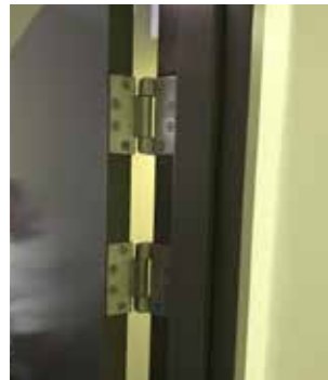
Figure 12.1 - Butt hinge
