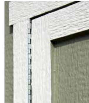
Figure 12.3 - Piano hinge
