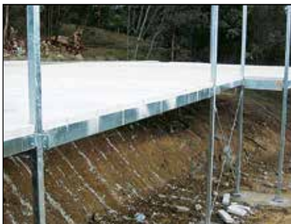
Fig 1.1 Residential Suspended Ground Floors
