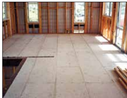
Fig 1.2 Residential Suspended First Floors
