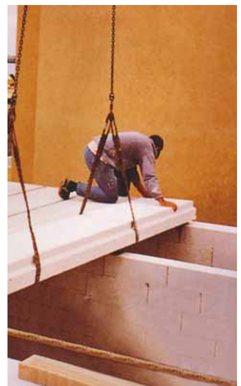
Image 7.3.3: Installing Floor Panels
