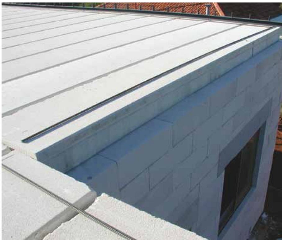
Image 7.3.2: Installed Floor Panels
