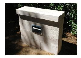
The capping blocks are laid flat and can overhang the front and rear of the wall for a great feature.
