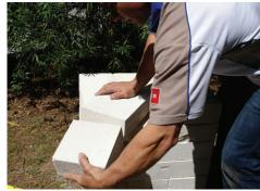
Cut 2 blocks to the width of the wall, and place these blocks at each end of the 3rd course as shown.
