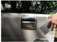
Fill the remaining 3rd course by cutting blocks to the required size to suit the gap either side of the letterbox. Use Hebel Adhesive on all block joins.
