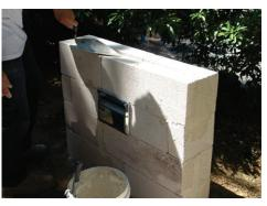
The fifth course is to "cap" the wall and cover the cavity between the front and rear walls.
