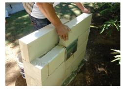
Apply Hebel Adhesive along the top of the third course and lay blocks for the fourth course, again, staggering the vertical joins between blocks to the course below.
