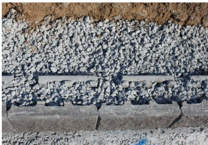
It is extremely important that bond be achieved between the wall units and the NFC. There is no point in building your Versawall® wall then filling up the void behind it with NFC afterwards. If you do this, the very first heavy rainfall event, where the water pushes through the voids in the NFC, will push over the wall units sitting in front of it.
