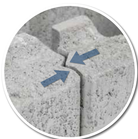
Interlocking tongue and groove joints
