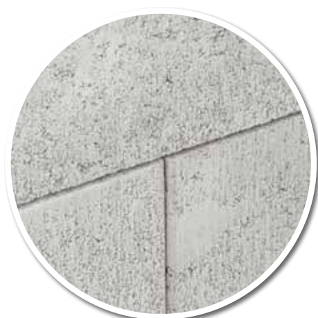
Clean wall with shadow lines
