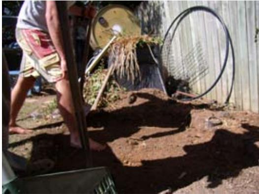
1. Your site must be level for good water distribution, so take time to prepare the foundation. Ensure that the site is level and free of deleterious material like roots and rocks.
