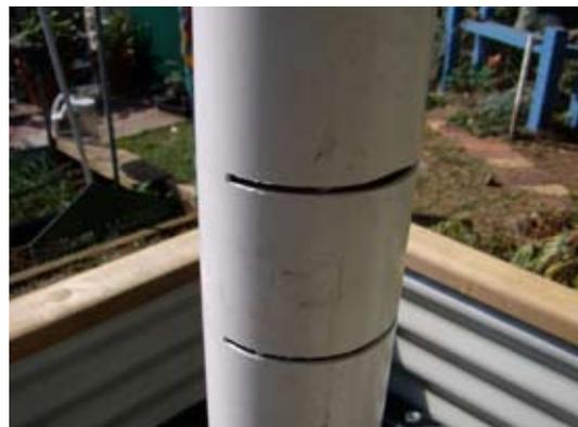
6. The slots of the filling tube face the base of the bed. This stops the coarse bedding sand back filling into the pipe, but allows water to exit the full length of the filling tube.
