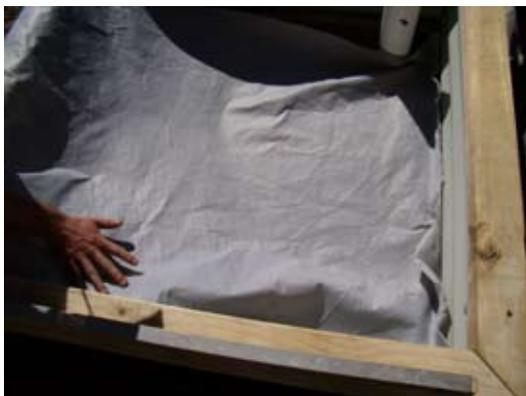
9. Place geo-textile fabric over the coarse bedding sand. This will prevent the soil media and bedding sand mixing.
