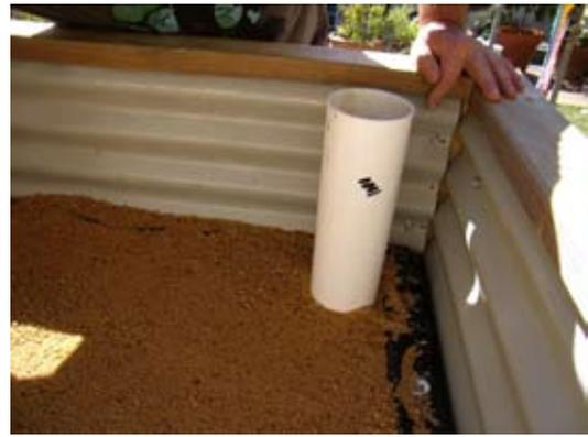
8. Gently spread and then screed the coarse bedding sand in and around the filler pipe **flat to the frame** of the reservoir. Do not compact this sand.
