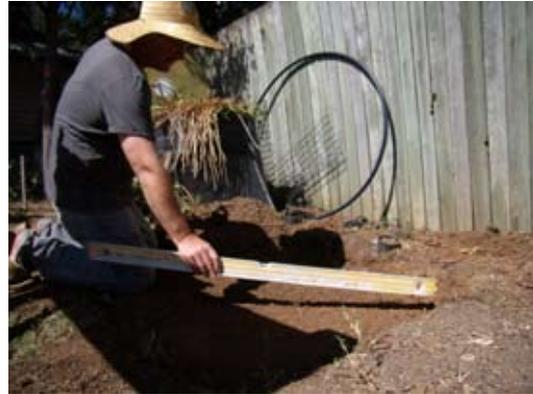
2. Spread a thin layer of coarse bedding sand over your prepared level site, this will prevent the membrane of the reservoir being punctured by anything unseen that is sharp.
