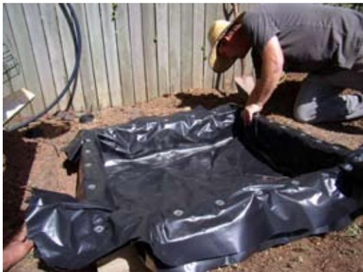
3. Set your reservoir assembly into position ensuring that the frame of the reservoir is level with only a slightest of fall to one side.
