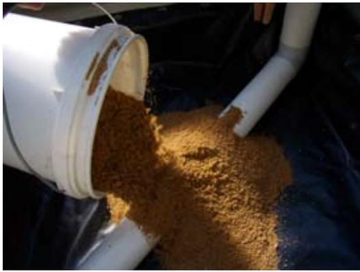
7. Add 200mm of coarse bedding sand to fill the reservoir void and create an aquifer.
