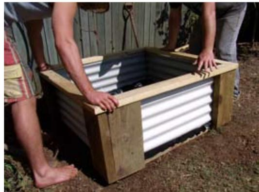
4. Slide the main raised garden frame over the reservoir section. This is a snug fit and should end up being absolutely level.
