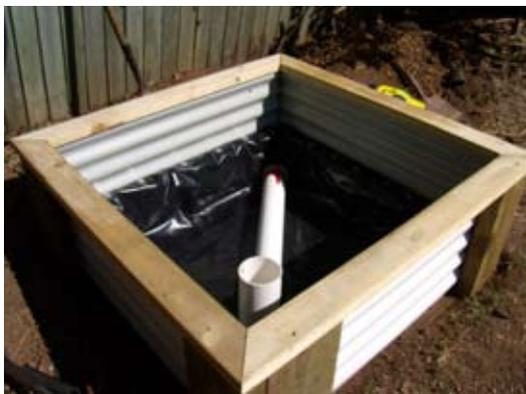
5. Place the filling tube in position across the bed, lying it on the black plastic liner. This should end-up being flat and level, so it will distribute the water across the bed evenly.
